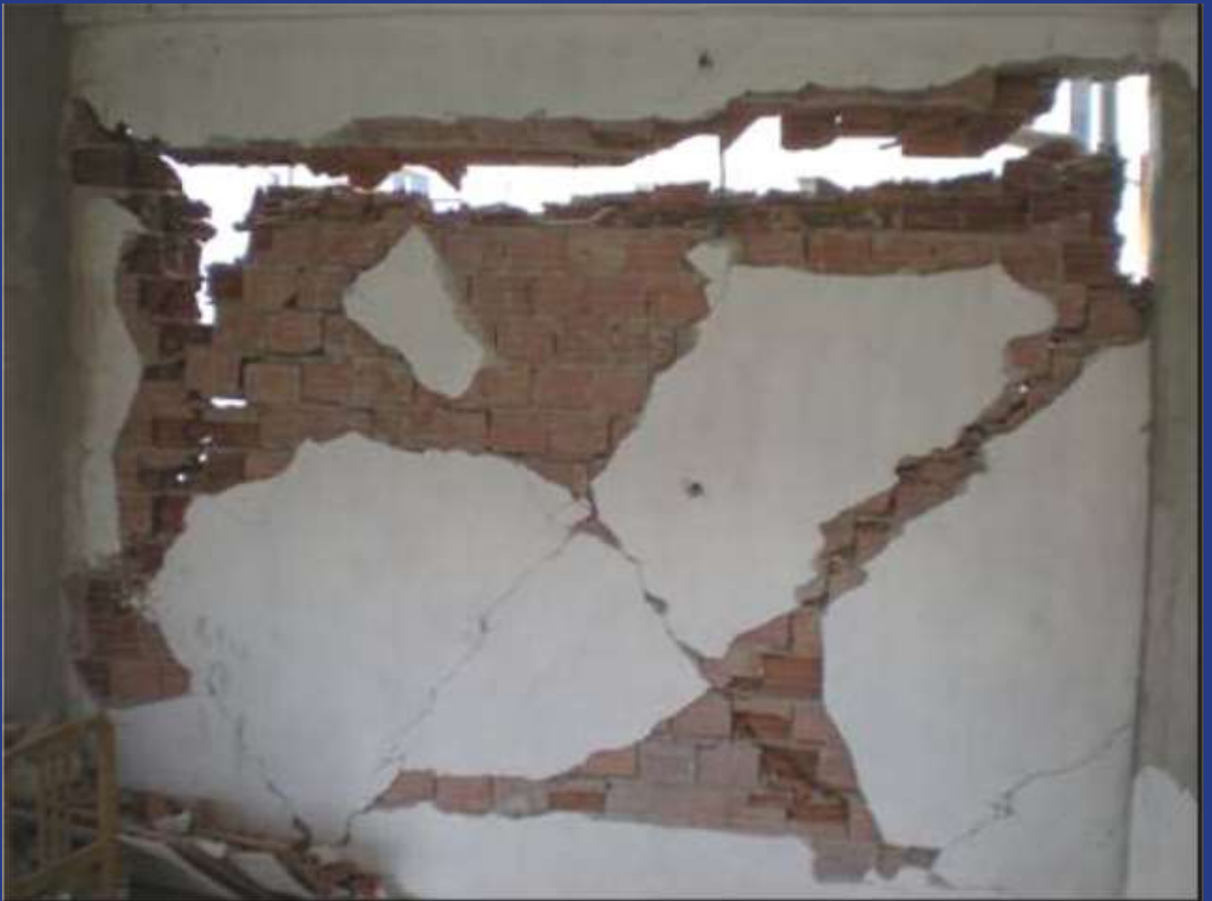
“X-shears” after an earthquake in Simav, Turkey!
