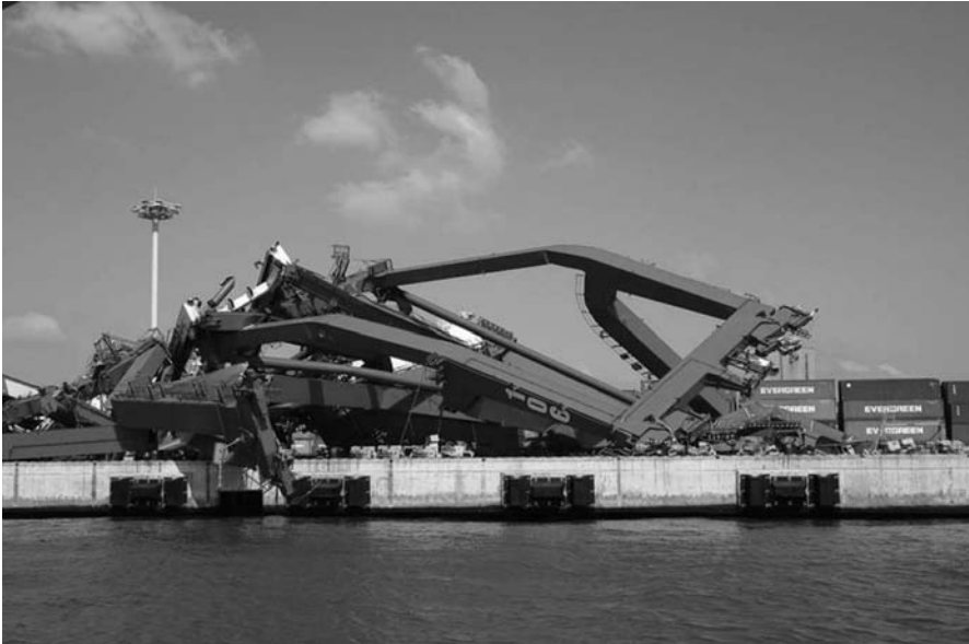
Fig. 11.1: Example of a port accident: crane collapse
